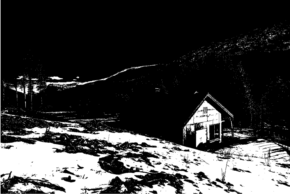
Picture 1: Setredalen Power Plant
