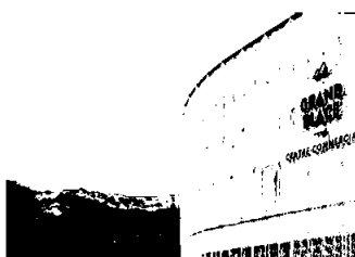
Grand Place Grenoble – France
