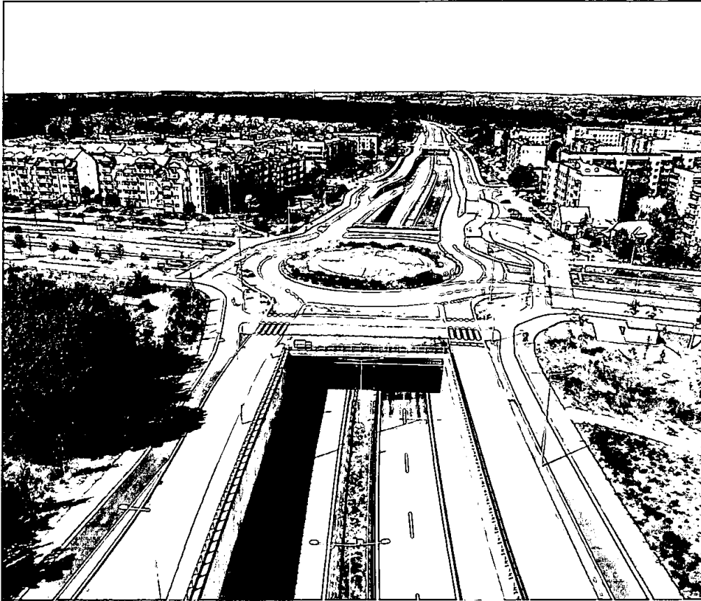
Bridge structures and retaining walls on the Trasa Niepodległości in Białystok, Poland
