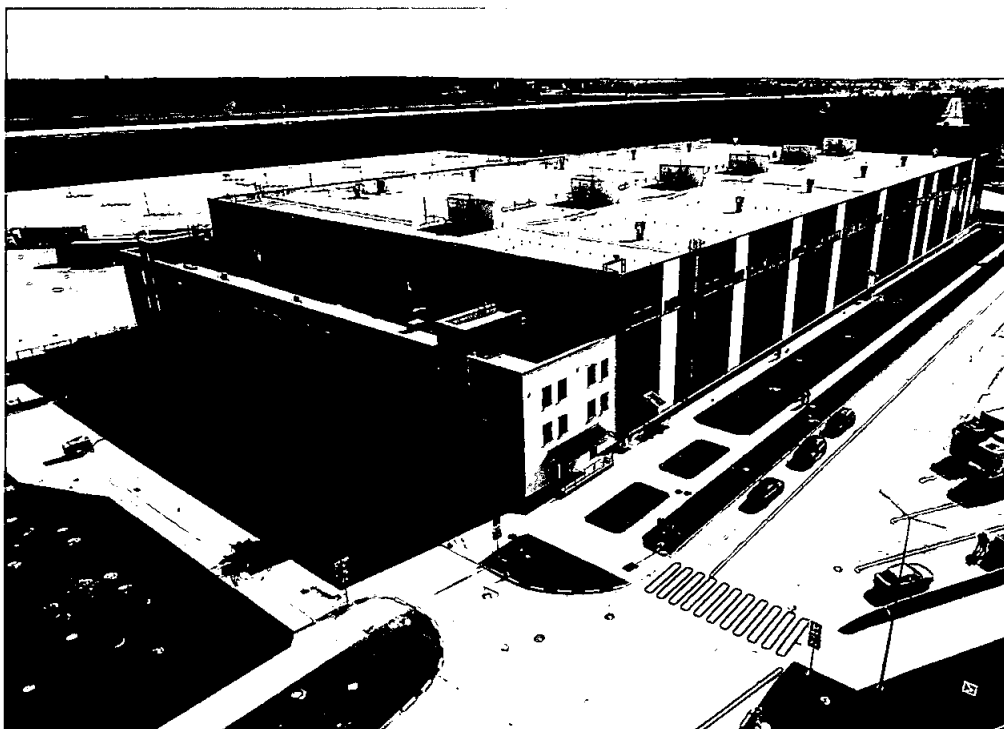
The "Bremino-Orsha" multimodal industrial and logistics complex in Bolbasovo, Belarus
