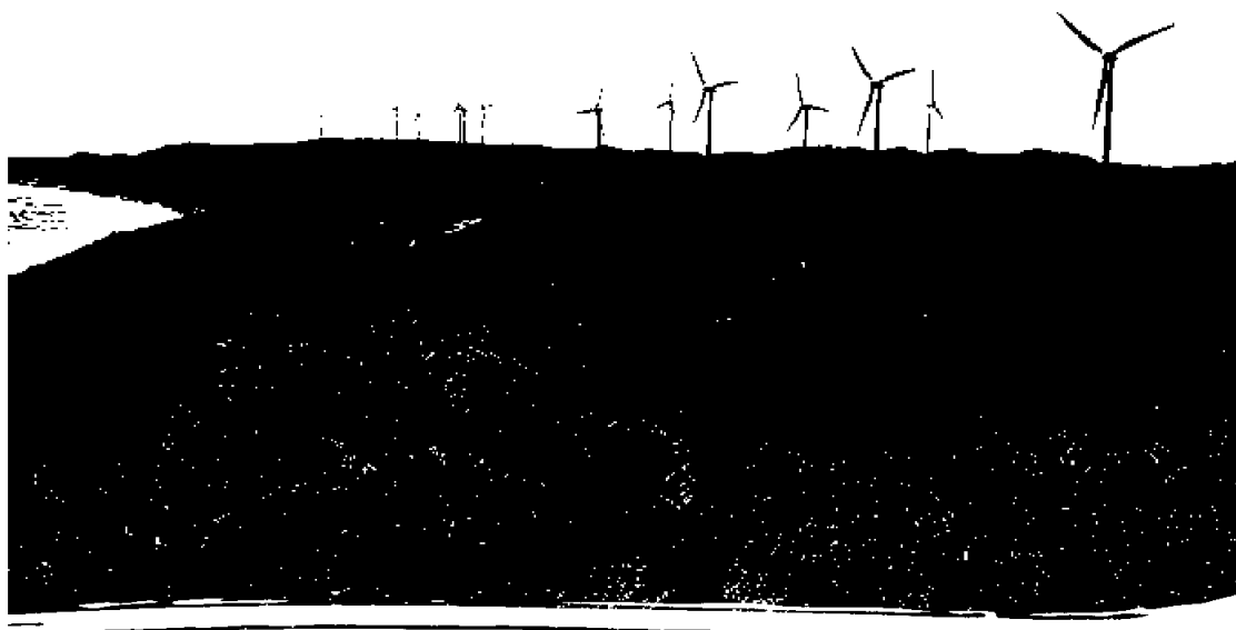
Albany Grasmere Wind Farm, for which Worley has been providing operations and maintenance services since 2018.
