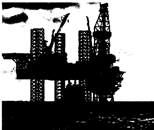
Angelin, Trinidad & Tobago Includes a new platform and four wells, with gas flowing to the Serrette platform hub via a new 13-mile pipeline.
