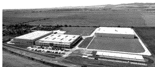
The Freudenberg Filtration Technologies plant in Potvorice, Slovakia, is one of the most modern in the Business Group's global production network.
